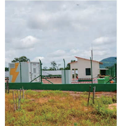
Telecom shelter project
