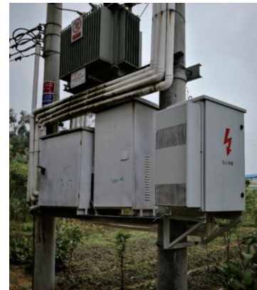
Southern Power Grid project
